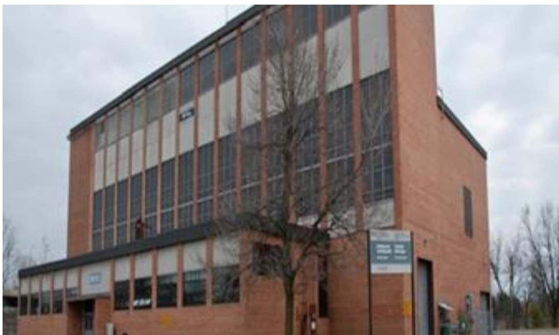
Confederation Heights Central Heating and Cooling Plant, Ottawa, Ontario, Canada. © Public Services and Procurement Canada (PSPC)
